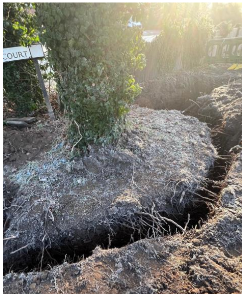
Examples of typical root damage caused by excavation works.
