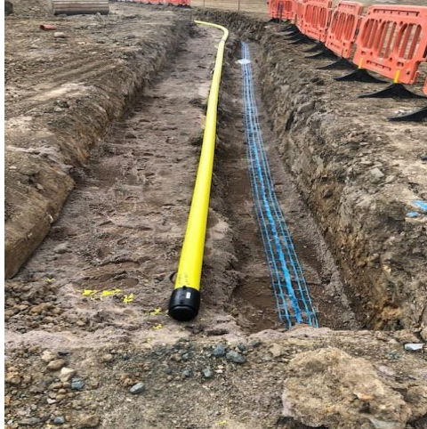
Figure 6 – Example of benching technique during multi-utility installation of gas and water
