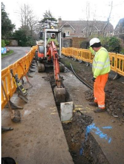
Additionally, lightweight service strike protection boards were designed and produced in conjunction with Pro-protect Safety Signs, and were issued to protect services that had already been exposed by safe digging.
