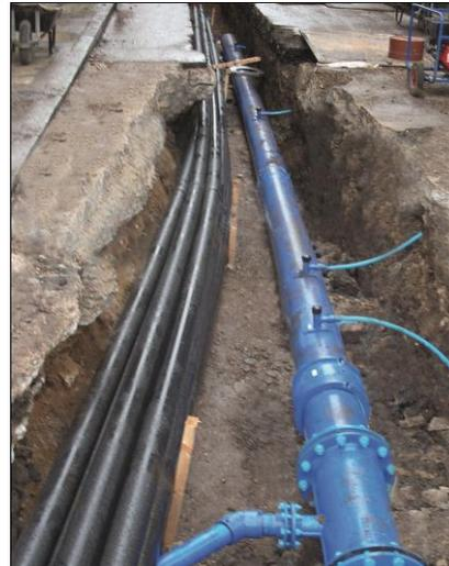
Just after work began in September 2009, UK Power Networks came to the table. They needed to lay approximately 200m of new 8-way cable power ducts to the Shard and it was agreed that Morrison Utility Services should also carry out this work in conjunction with the gas and water main projects.
