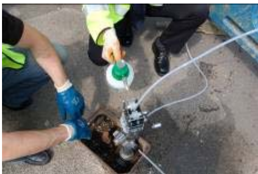
Live Camera Inspection
