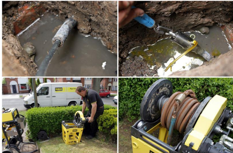
The Kobus pipe puller in action
